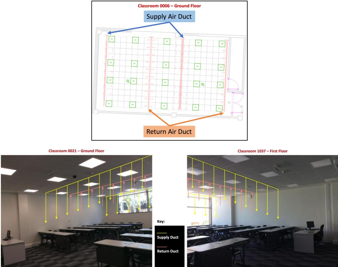
Figure 20: Showing the Supply and Return Air Ducts in Three Classrooms
