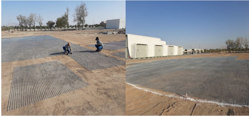
Figure 13: Preparation of steel mesh floor at UAEU Radio-array site
