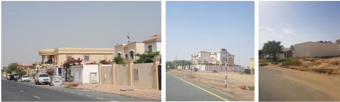
Figure 32: Inadequate Accessibility of Streets in Al Khawaneej First, taken by author (2018)
