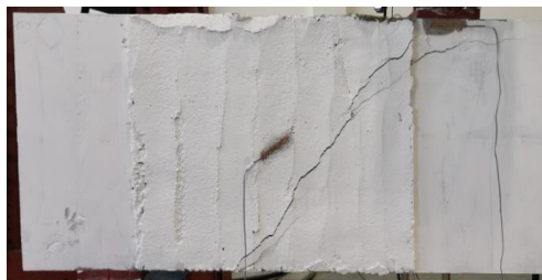
Figure 4.7: Crack pattern of specimen NS-C1-90: A. Schematic drawing of the crack pattern, B. Picture of the beam at failure, C. Close view of the crack pattern (west shear span)
