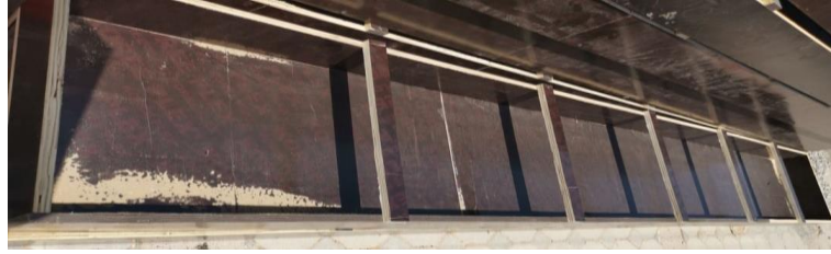
Figure 3.7: Formwork of the beams
