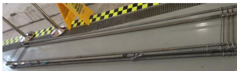
Figure 3.6: Steel cages of the beams without stirrups
