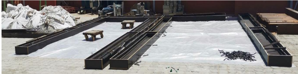
Figure 3.11: Steel cages inside the forms
