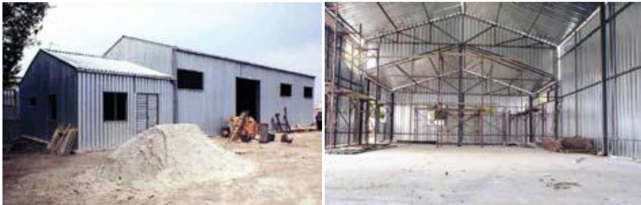
Figure 7. All-metal workshop under construction. (Sciortino & FAO, 2010).
