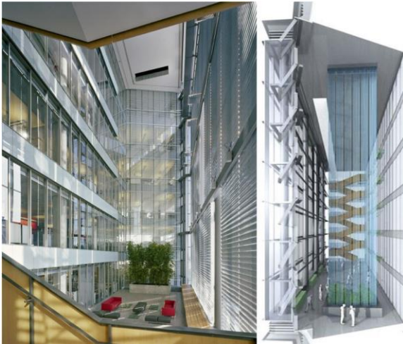
Figure 13. The water feature used to condition the internal air in both summer and winter ( https://www.kpmb.com/project/manitoba-hydro-place/ )
