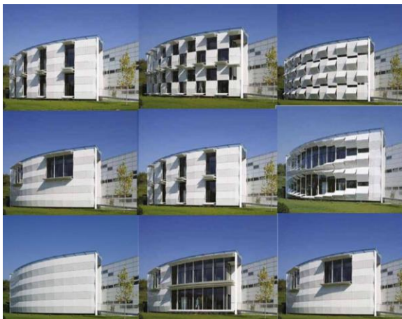
Figure 7. kiefer technic showroom dynamic envelope.
