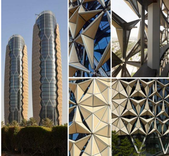
Figure 9. Al-Bahr Tower exterior adaptive façade external and internal shots (different websites)
