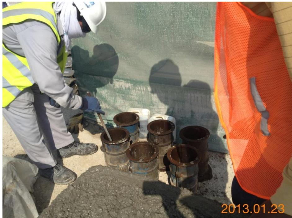
Figure 3.9: Preparation of concrete cylinder samples
