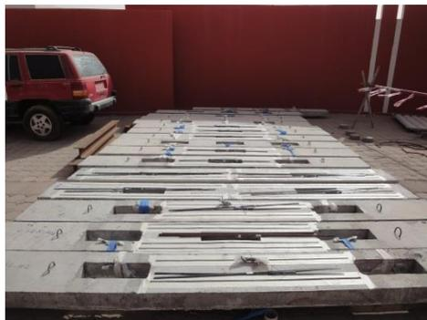
(e) Installation of CFRP strips
