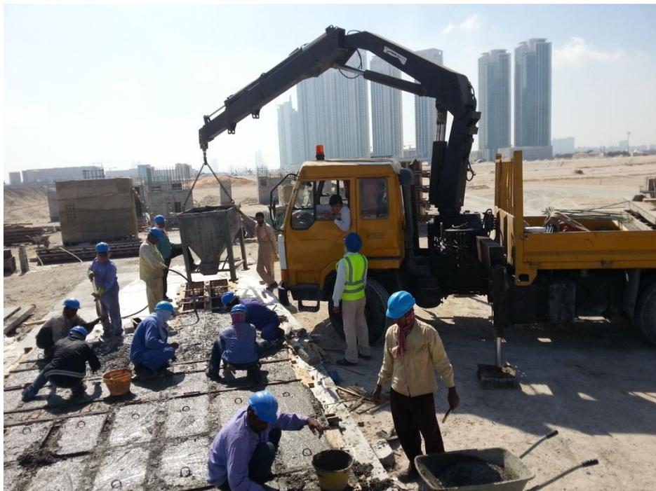
Figure 3.7: Concrete casting
