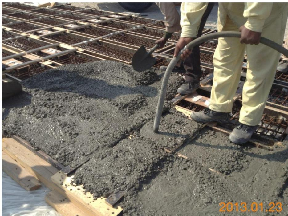
Figure 3.8: Concrete vibration
