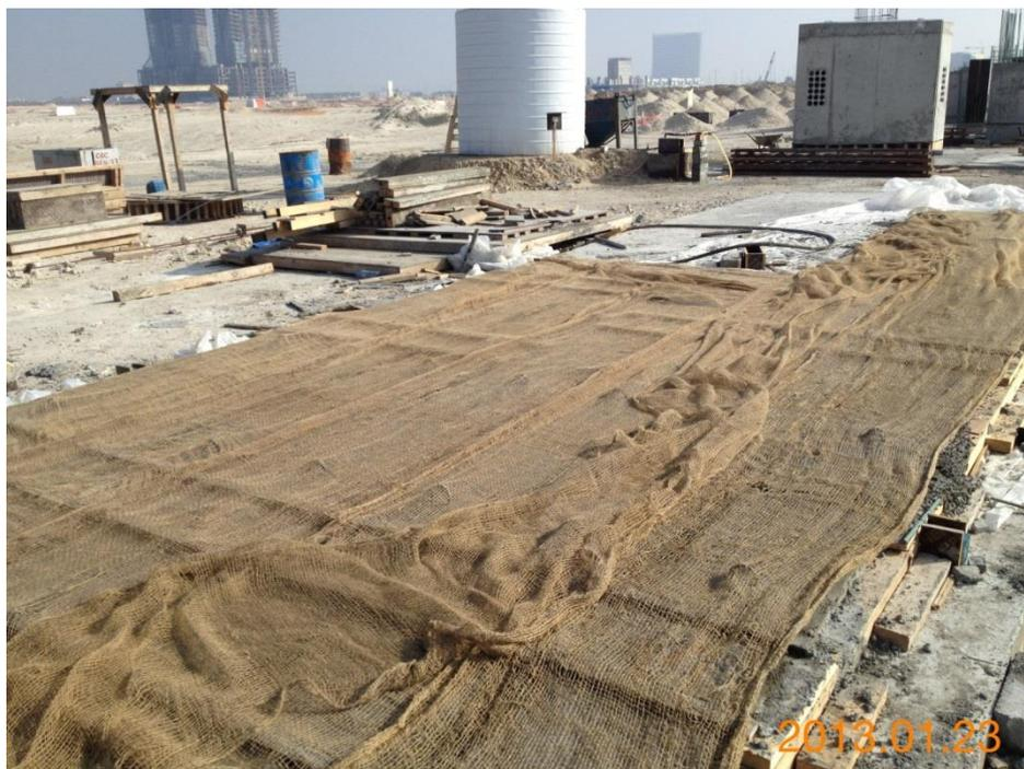
Figure 3.11: Concrete curing
