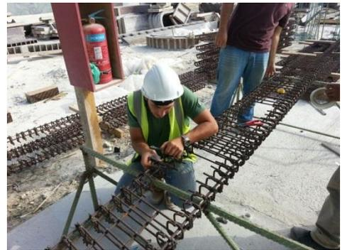
(b) Cleaning of steel surface by alcohol
