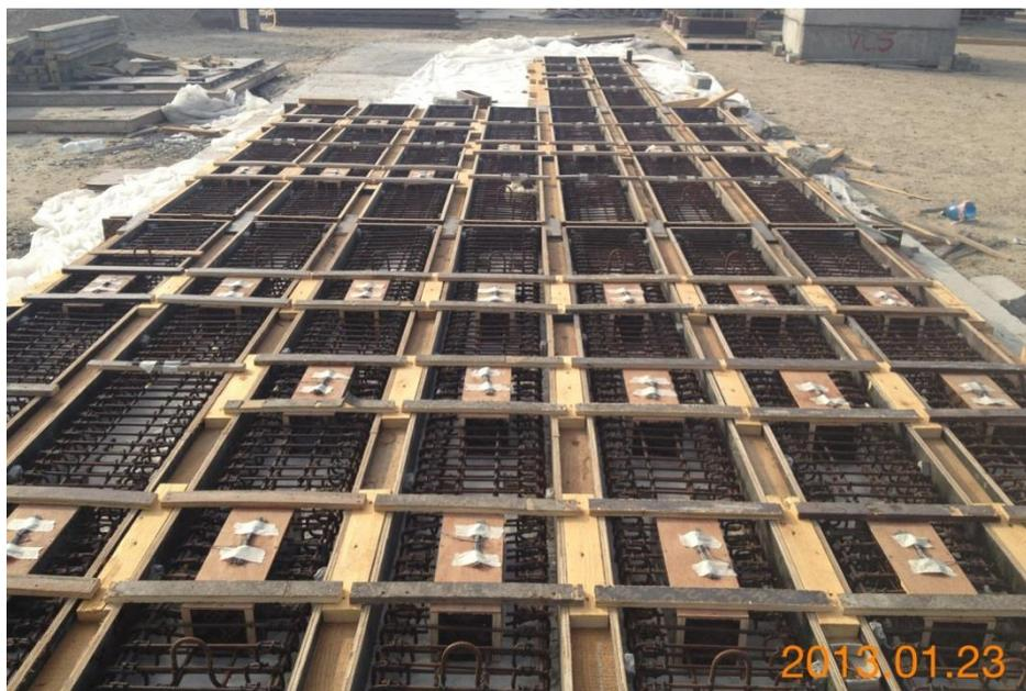
Figure 3.6: Steel cages installed inside the forms
