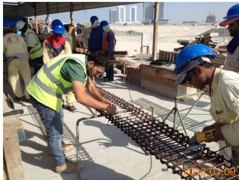
(a) Surface preparation using grinder
