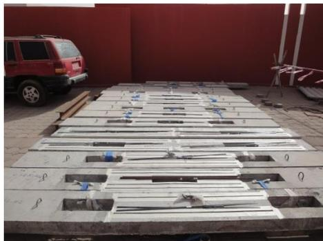
(e) Installation of CFRP strips
