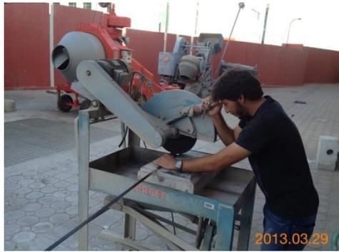
(a) Cutting of CFRP strips
