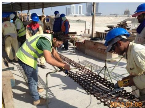
(a) Surface preparation using grinder
