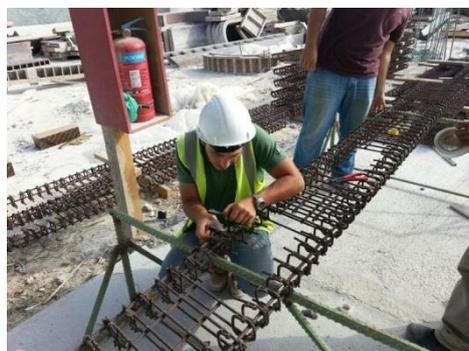
(b) Cleaning of steel surface by alcohol
